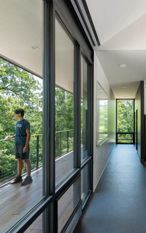
The porch is an important component to any architype in the area, whether it be for informal meeting, relaxing, or taking in the view. The back porch is elevated and cantilevered into the tree canopy. The space is intentionally column free to allow unobstructed views into the trees and surrounding site. The overhang above the porch also shades the larger expanses of glass into the main common area. Shadows and textures of the tree canopies dance across this space throughout the day.
