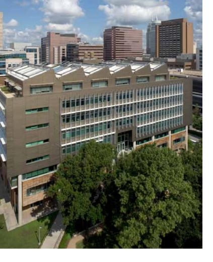
Because of the limits of the available site, the building is oriented with its long axis in a north-south direction. A breezeway connection—a two story open air space carved from the lower levels of the building—runs east to west allowing the entrance and the main public spaces to be oriented toward Fay Park. Each façade of the building was designed with unique fenestration and sun screening strategies, all of which were computer modeled by BNIM to maximize building performance.
